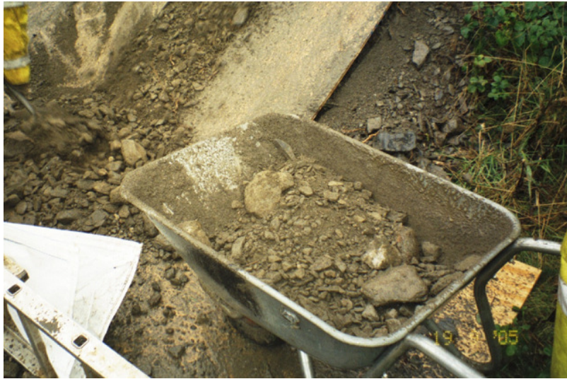
Figure 3: Sample of glacial till used for shoulder fill
